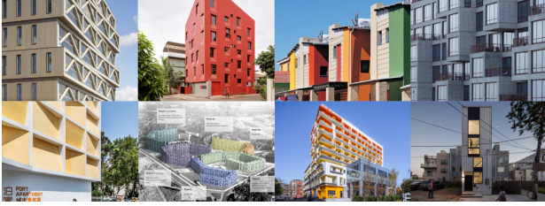
Figure 1. Selected contemporary case studies. From left (top) to the right (bottom): PATCH 22 (Amsterdam), Stacked student housing (India), 10x10 affordable housing (South Africa), 222 Jackson Avenue (USA), Yuntai apartment complex (China), Beton student housing (UK), Xizhimen apartments (China), Tiny tower (USA).
