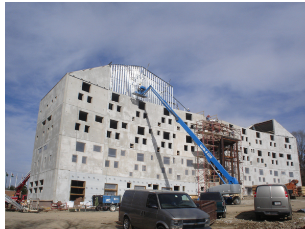
Figure 3: Pre-cast concrete structure. Source: (Author 2006)
