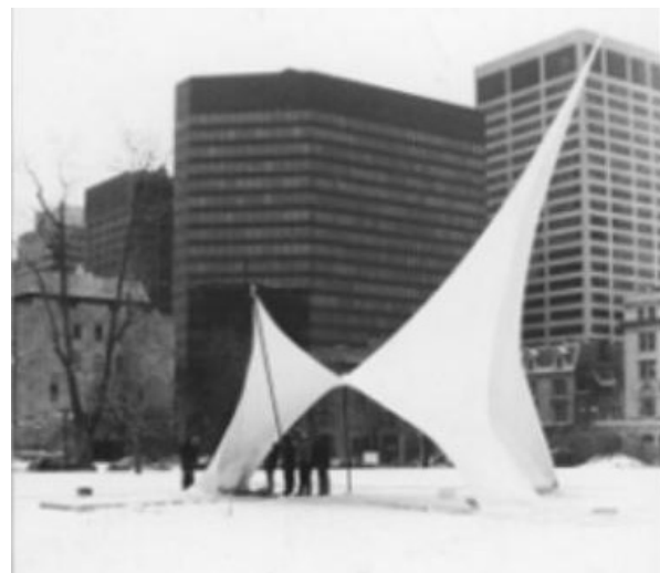
Figure 8: Nylon-reinforced, double-curved ice structure with free edges
