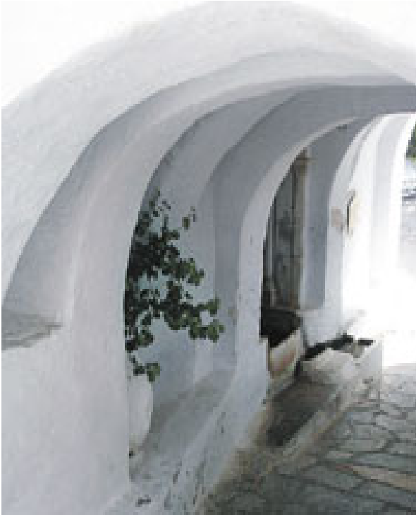
Figure 6: Spaces protected from the intense solar radiation with manufactures that are parts of the buildings. Source: (author, 2000)
