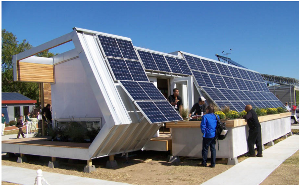
Figure 5. South and west elevations, Project Solar House. Note the form has been canted to maximize solar production. Source: (Gabbard 2007).
