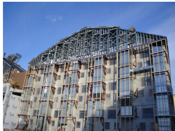
Figure 4: Pre-cast concrete structure with return air stacks during rough framing. Source: (Author 2006)
