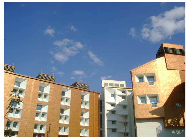
Figure 8: Stack exhaust termini types. Source: (Author 2007)
