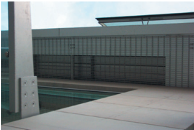
Winter Wall Section: Dampers Closed
