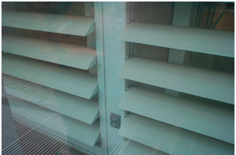
It can be seen that the louvers are fixed in a horizontal position, painted white and are very dirty.
