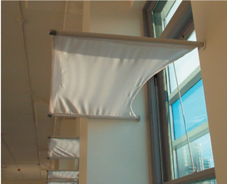
A view of the shading device attached to the interior of the windows. It also serves as a daylight reflector/light shelf to bounce light up to the white painted concrete ceilings.
