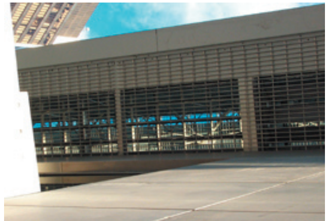
Summer Wall Section: Dampers Open
